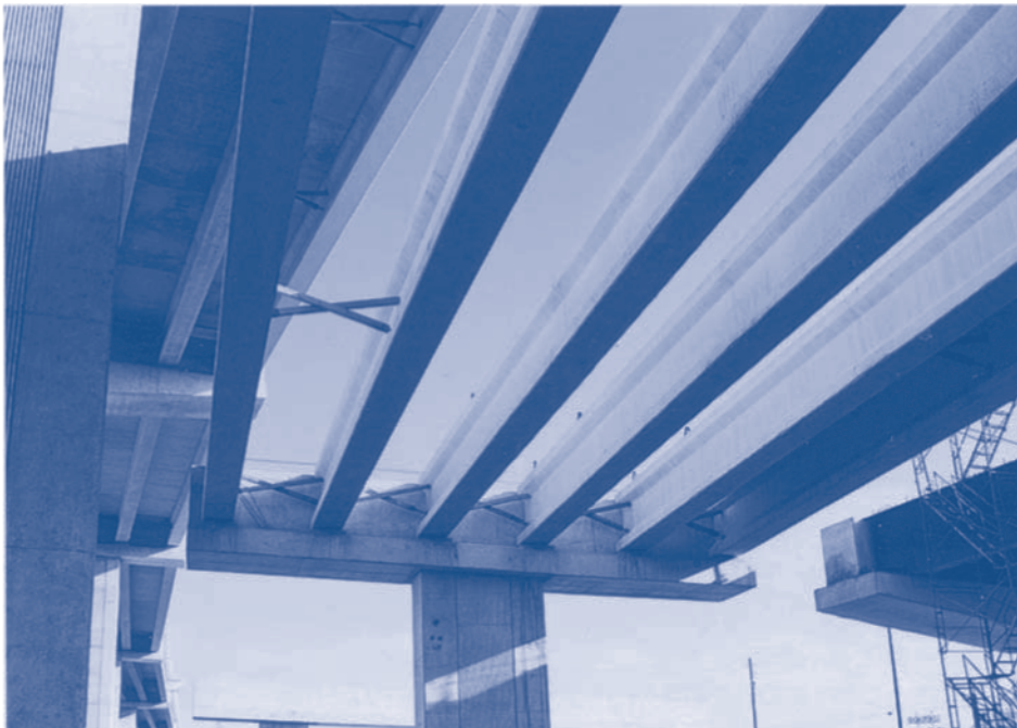
FIGURE 5.1 Several bridge beams during bridge construction. (Courtesy Roy Craig)
