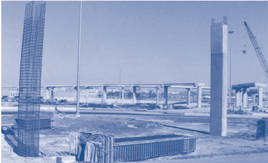
FIGURE 3.1 Some reinforced concrete columns for highway interchange bridges. (Courtesy Roy Craig)
